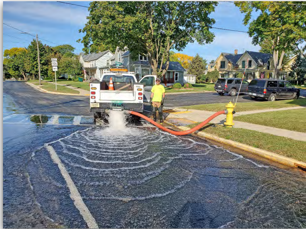
DAN SCHIENLEBER FLUSHES HYDRANTS IN OCTOBER AT THE CORNER OF ADAMS ST. AND SHERMAN AVE. W.
