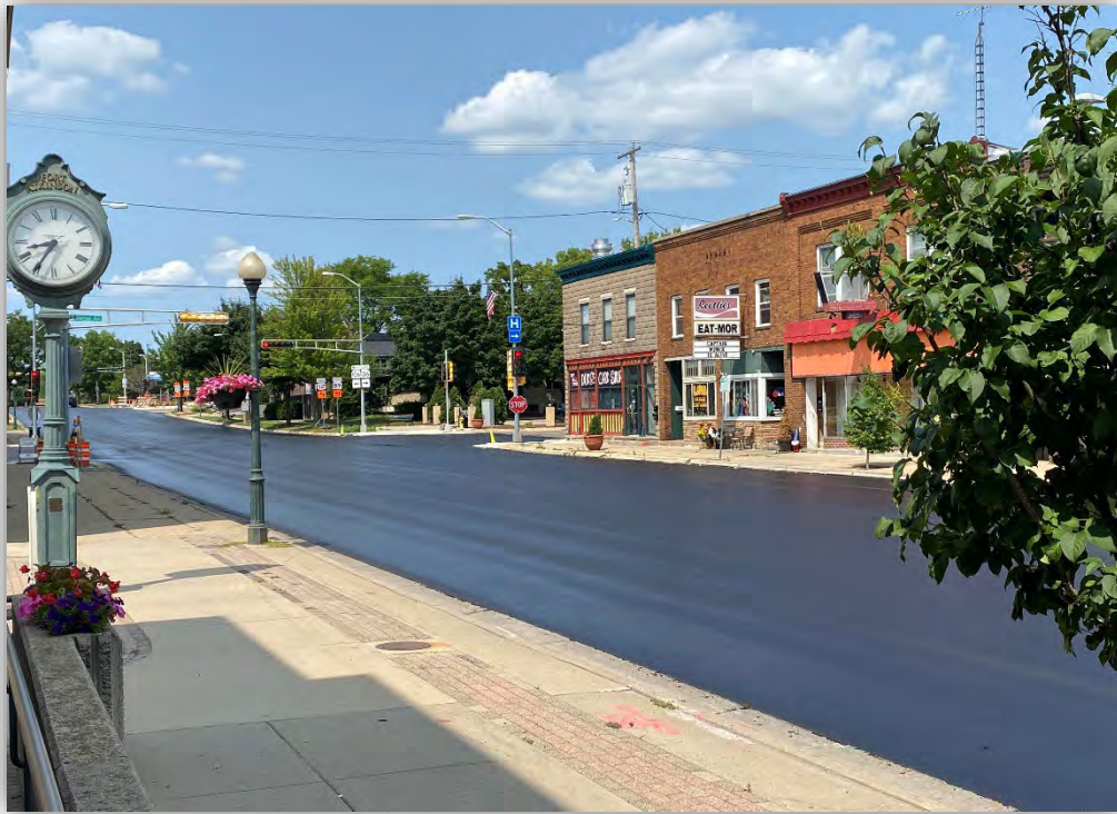
NORTH MAIN STREET IS SEEN SHORTLY AFTER PAVING AUG. 1.
