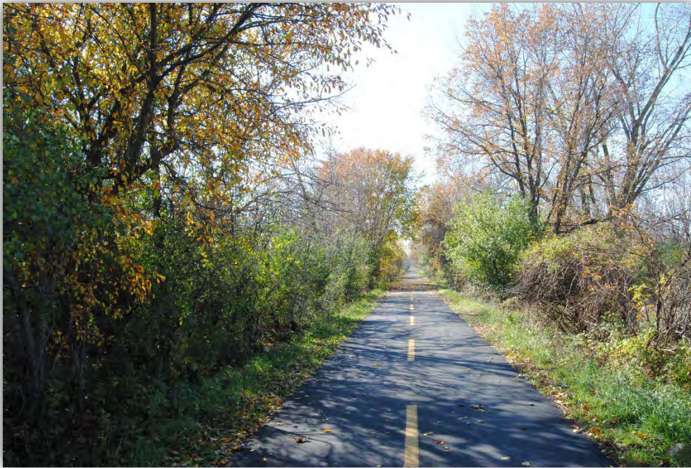
A PORTION OF THE BIKE TRAIL IS SEEN NEAR THE WASTEWATER TREATMENT PLANT.
