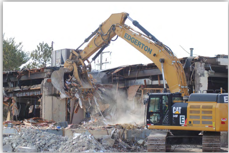
THE DEMOLITION OF THE LORMAN SITE IS SEEN IN NOVEMBER 2022.
